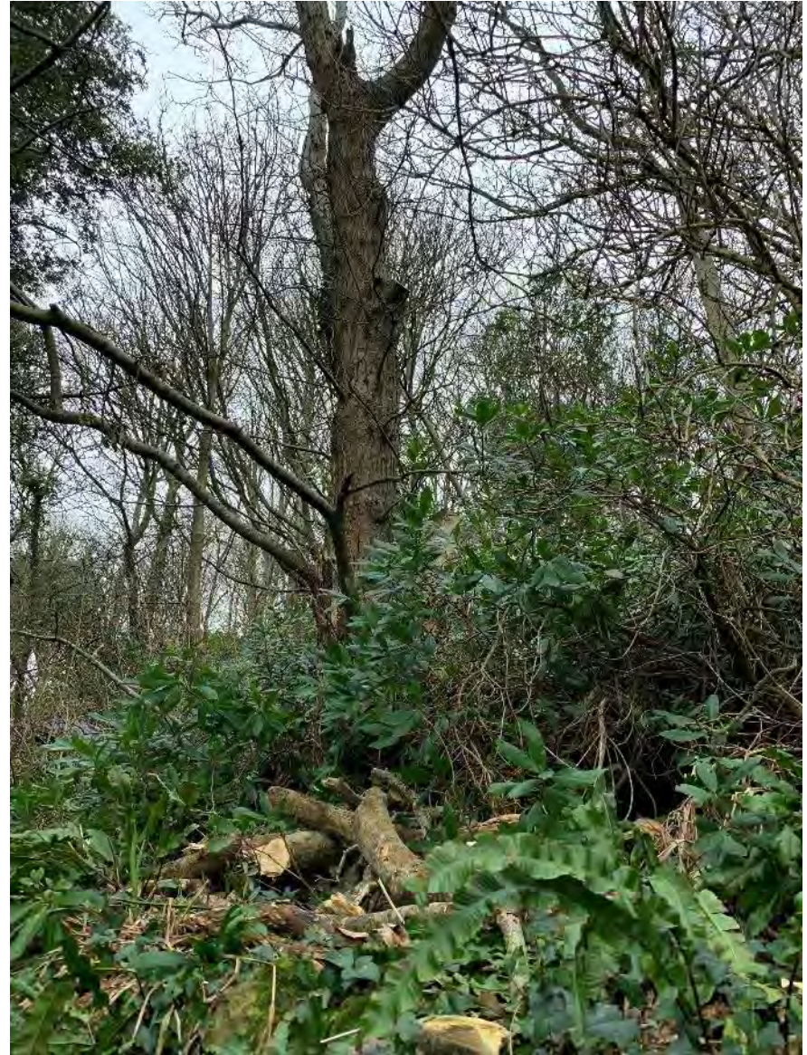
Line 52 IOW_4_S026 to S028/Tree Works
