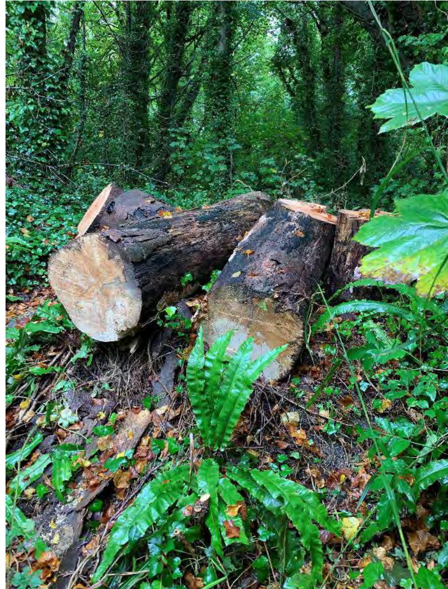
Line 48 IOW_4_S010 to 018/ Tree Works (1)
