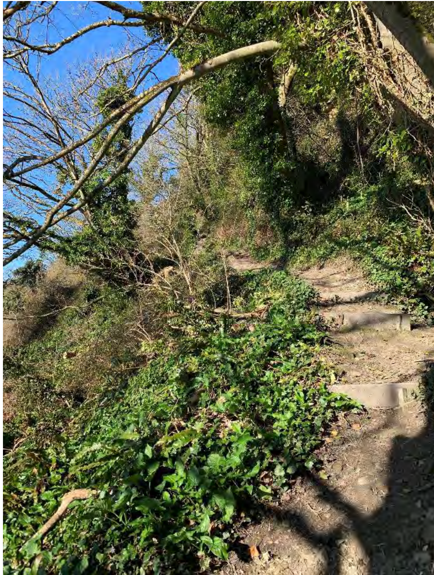
Line 54 IOW_4_S050/Tree Works
